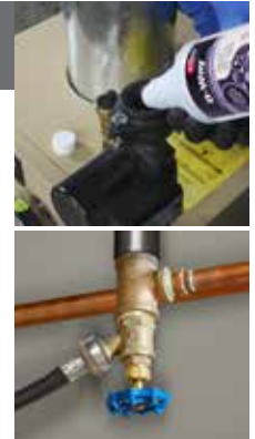
▲ Force pump drain line injection
